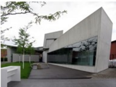
Vitra Fire Station in Weil am Rhein, Germany (1991-93)
